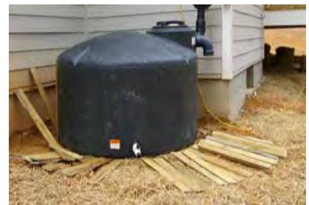
Natural systems collect and treat storm water runoff; Rain barrels collect storm water runoff and store for reuse.
