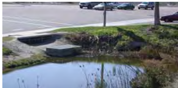
Detention basin used to allow pollutants to settle instead of draining directly into the lagoon
