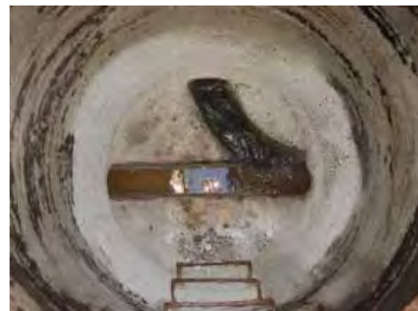
Interior of a sanitary sewer manhole
