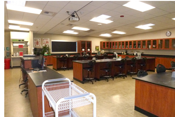
(Top) Chemistry labs in building 4500 have mechanical fume hood issues and do not support 21st century learning.
