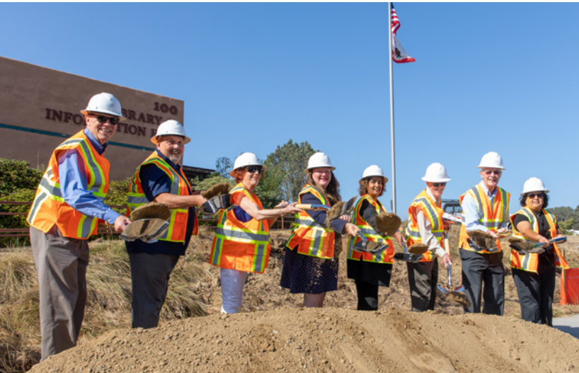
Groundbreaking of new Student Services and Administration Building at the San Elijo Campus
