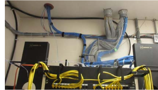
Figure 2 – IDF in building 4600.
