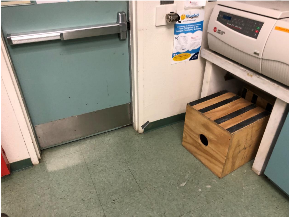
Photo 11 – Building 400 / Room 402, 4" Vinyl Cove Base (Light Green) w/ Adhesive.
