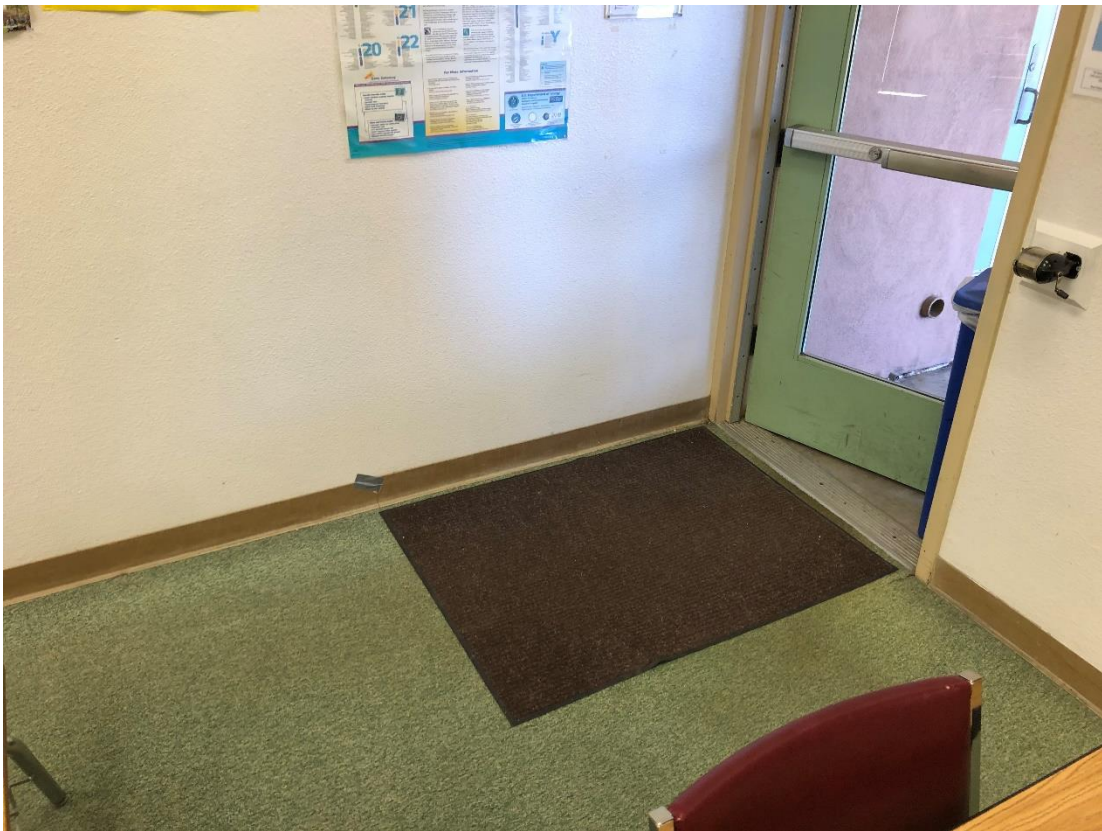
Photo 12 – Building 400 / Room 401, 4" Vinyl Cove Base (Tan) w/ Adhesive.
