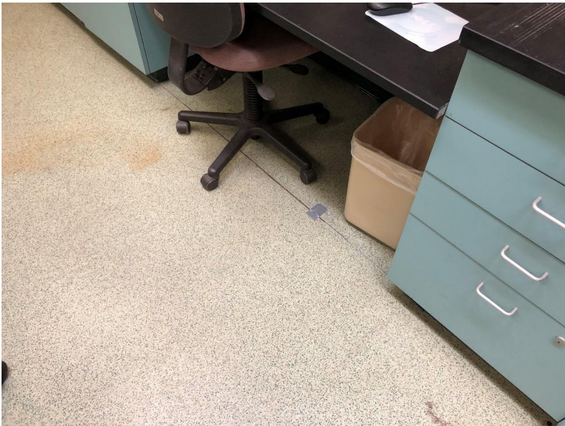
Photo 8 – Building 400 / Room 404, Vinyl Sheet Flooring (Green Speck) w/ Mastic
