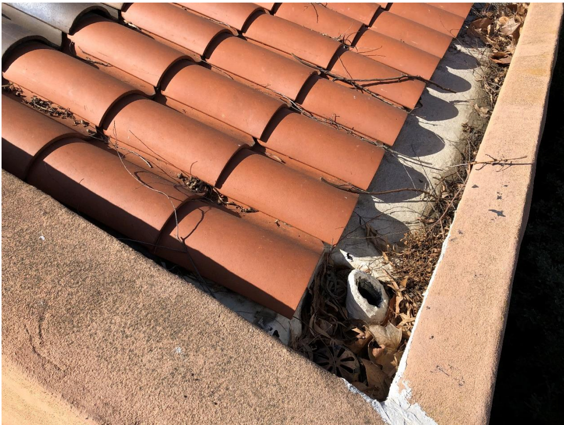
Photo 18 – Building 400 / Exterior East Tile Roof, Roofing Sealant (White)/ Roofing Mastic (Black).
