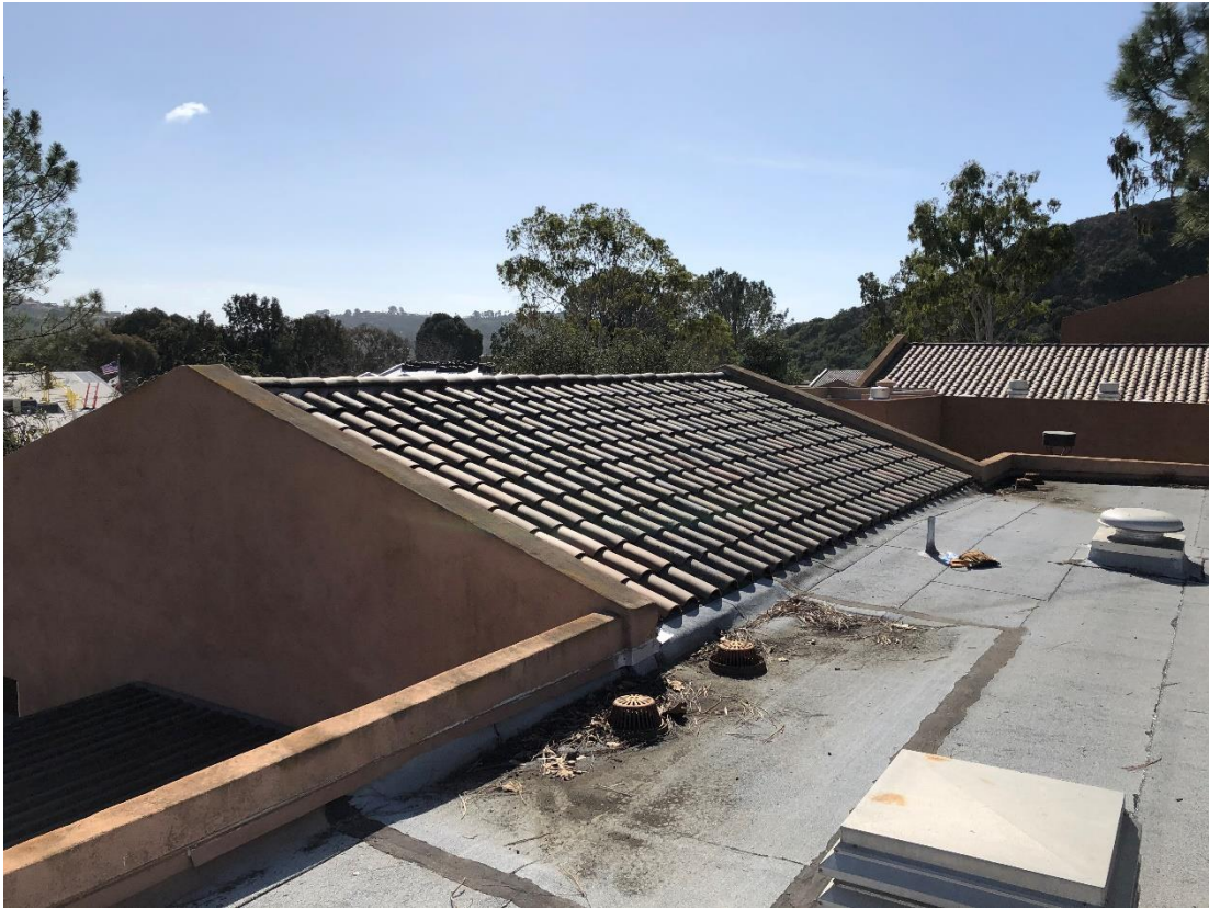
Photo 17 – Building 400 / Exterior SW Tile Roof, Roofing Felt under Tiles.
