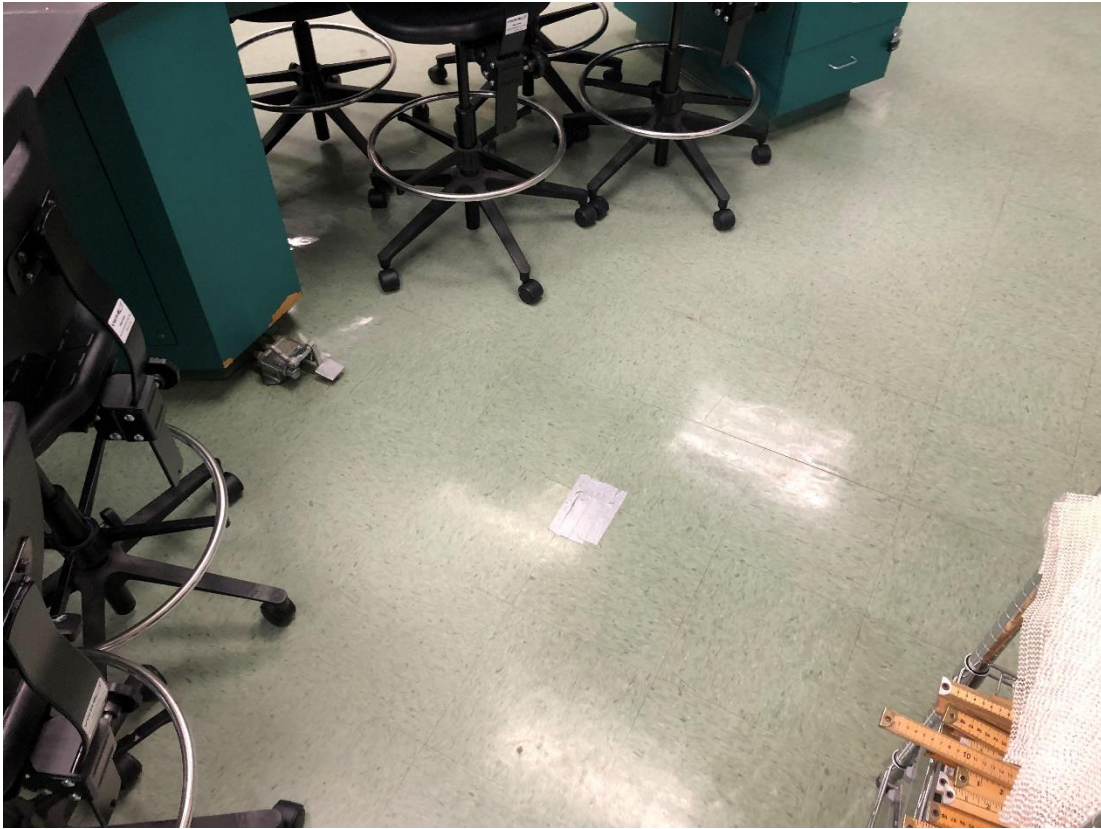
Photo 19 – Building 400 / Room 402, Concrete Slab under Vinyl Floor Tile.
