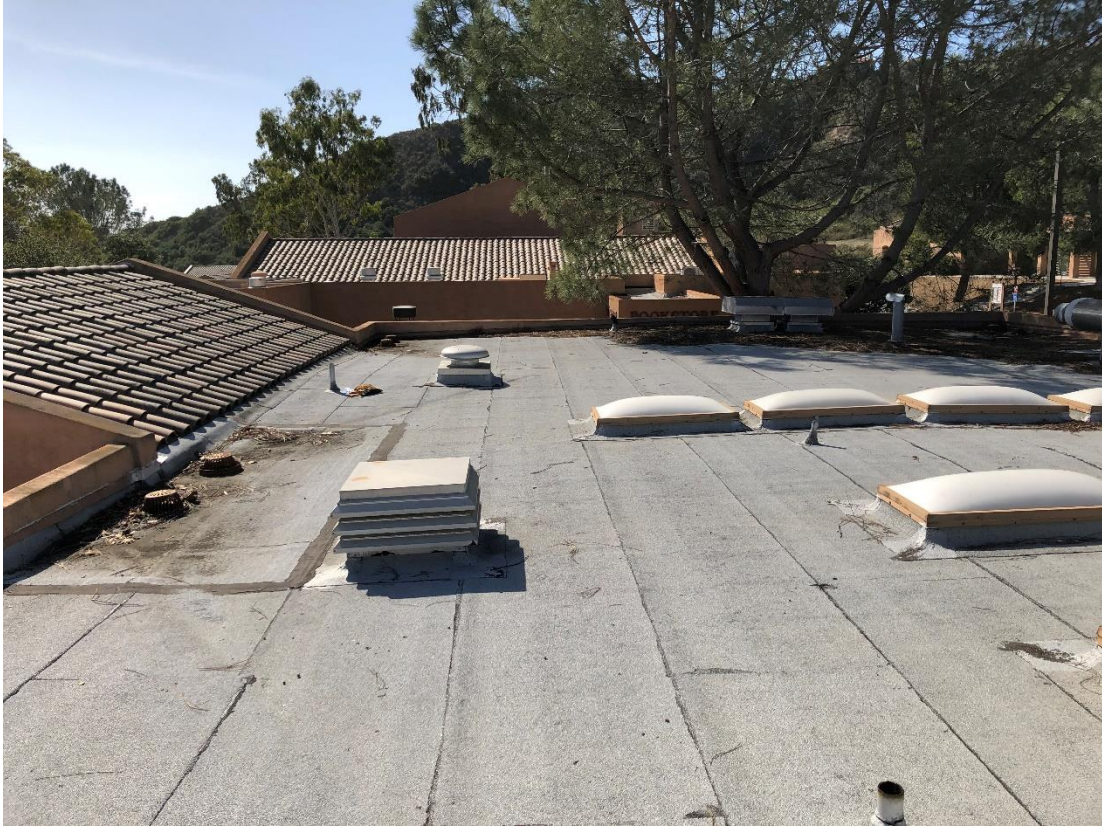
Photo 15 – Building 400 / Exterior Main Roof, Built-up Roofing Material.
