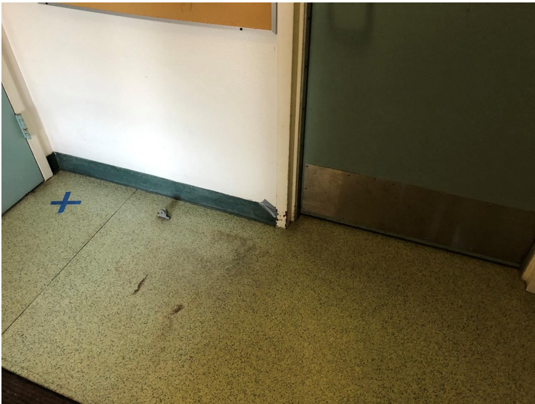
Photo 10 – Building 400 / Room 402B, 4" Vinyl Cove Base (Dark Green) w/ Adhesive.
