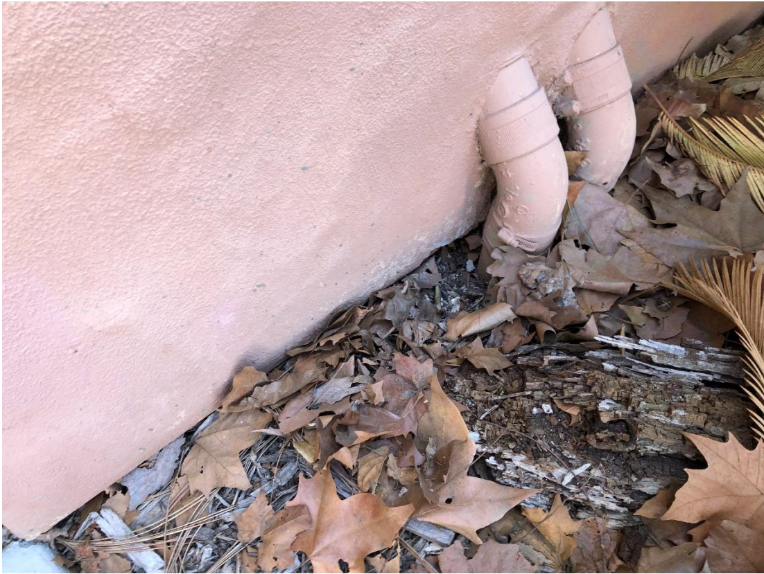
Photo 13 – Building 400 / Exterior, Stucco at North Wall New West Door Proposal.
