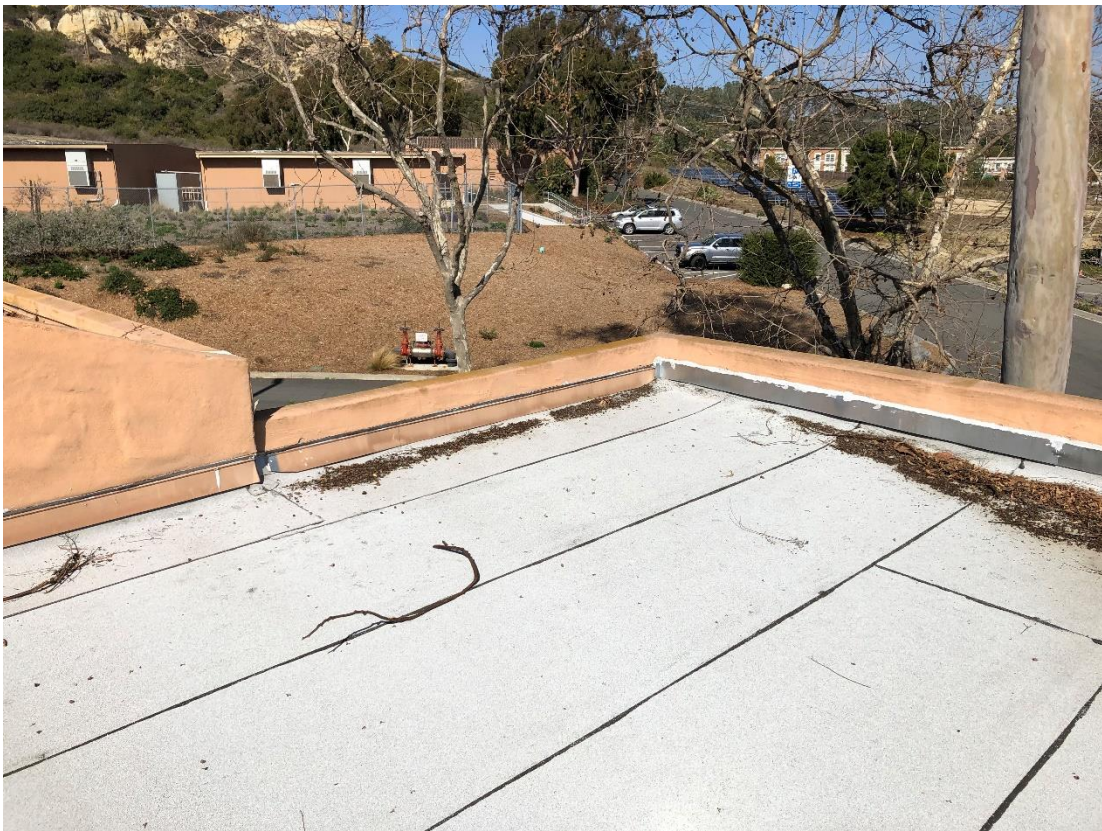
Photo 14 – Building 400 / Exterior SE Roof, Stucco at NE Parapet.
