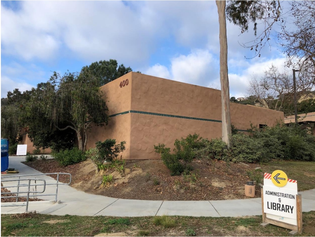
Photo 1 – MiraCosta College San Elijo Campus Building 400, located at 3333 Manchester Ave., Cardiff, CA.
