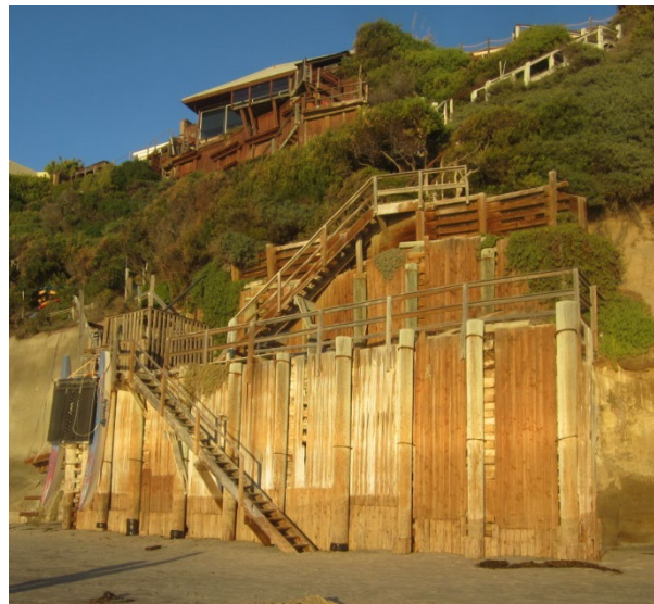
Telephone Pole Seawall
